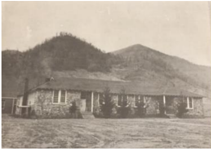
The Maggie Valley School was built in 1930. It had four rooms to replace several one-room schoolhouses
